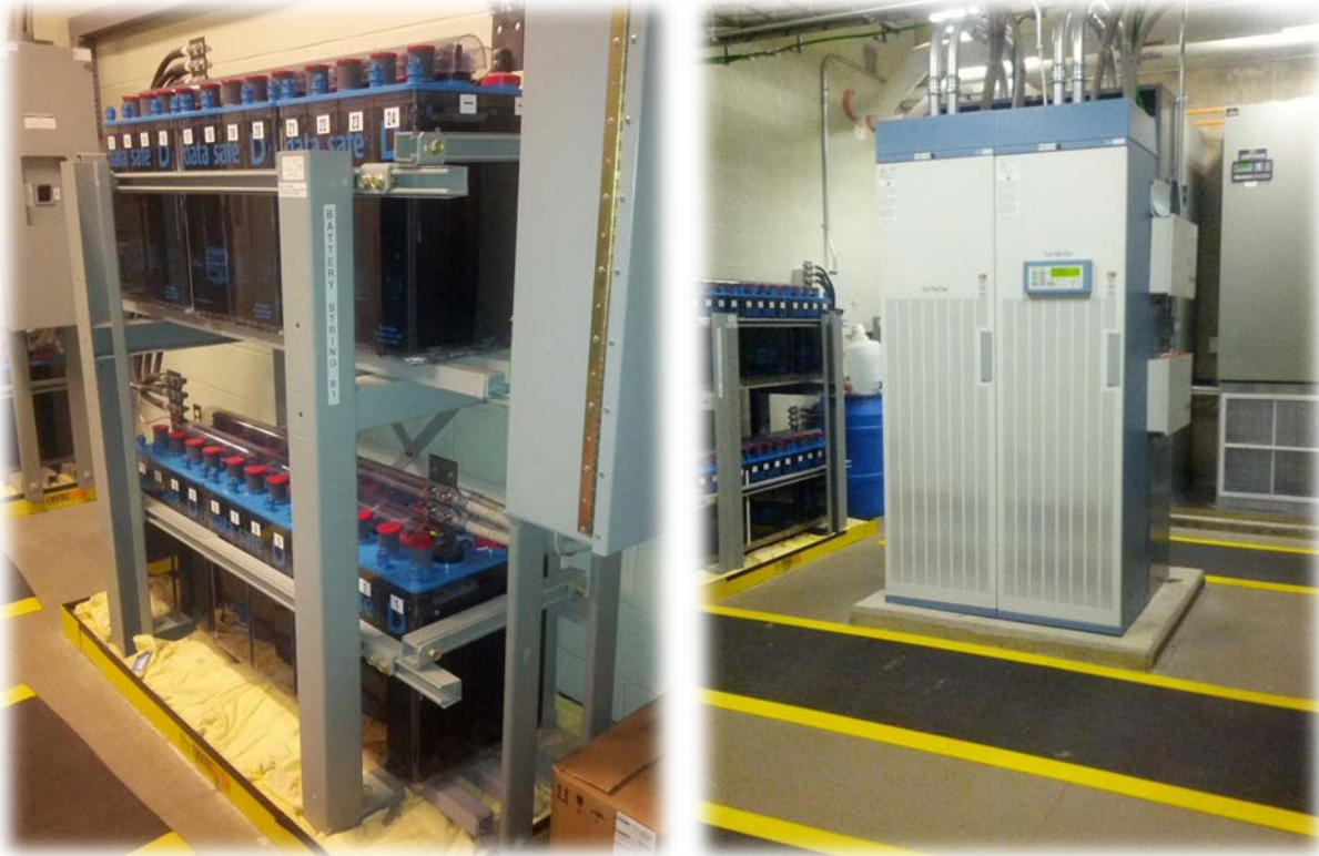
Part of the DC power plant working on batteries
